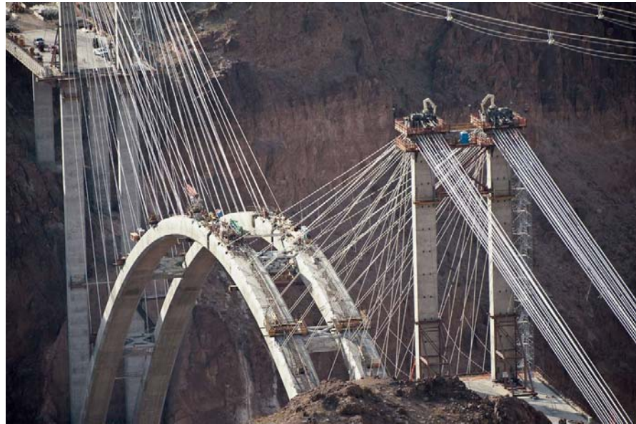
Construction of arch piers
