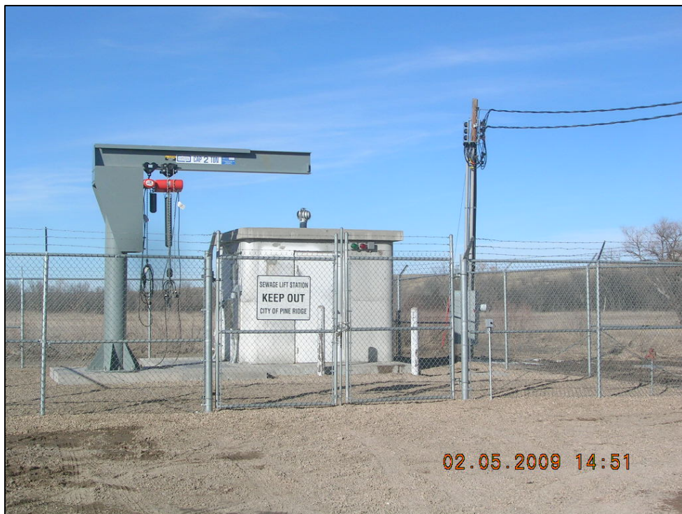
Completed Renovation of the Pine Ridge Sewage Lift Station.
