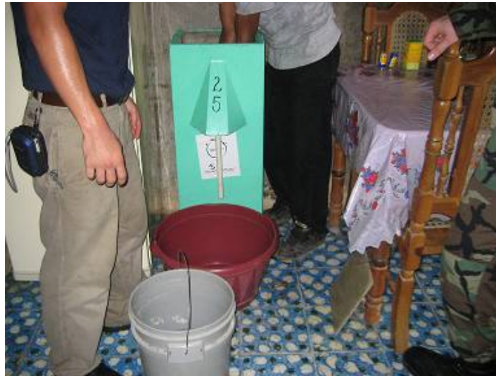
Installation of BSF Unit in Codigo
